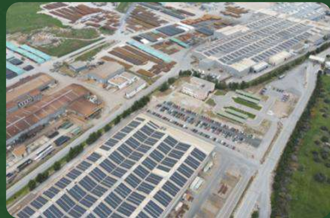
Corinth Pipeworks Factory (VIOCHALKO group) 7.100KWp The largest PV on industrial roof in Greece
