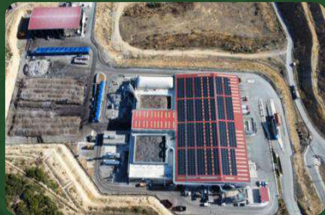
Waste Treatment Unit (WTP) of Alexandroupolis 700KWp + 200KWh storage (BESS)
